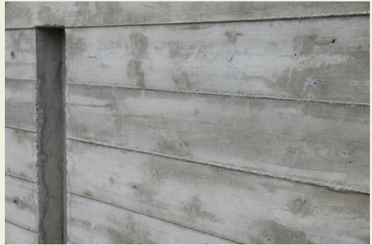
Board Formed Concrete
