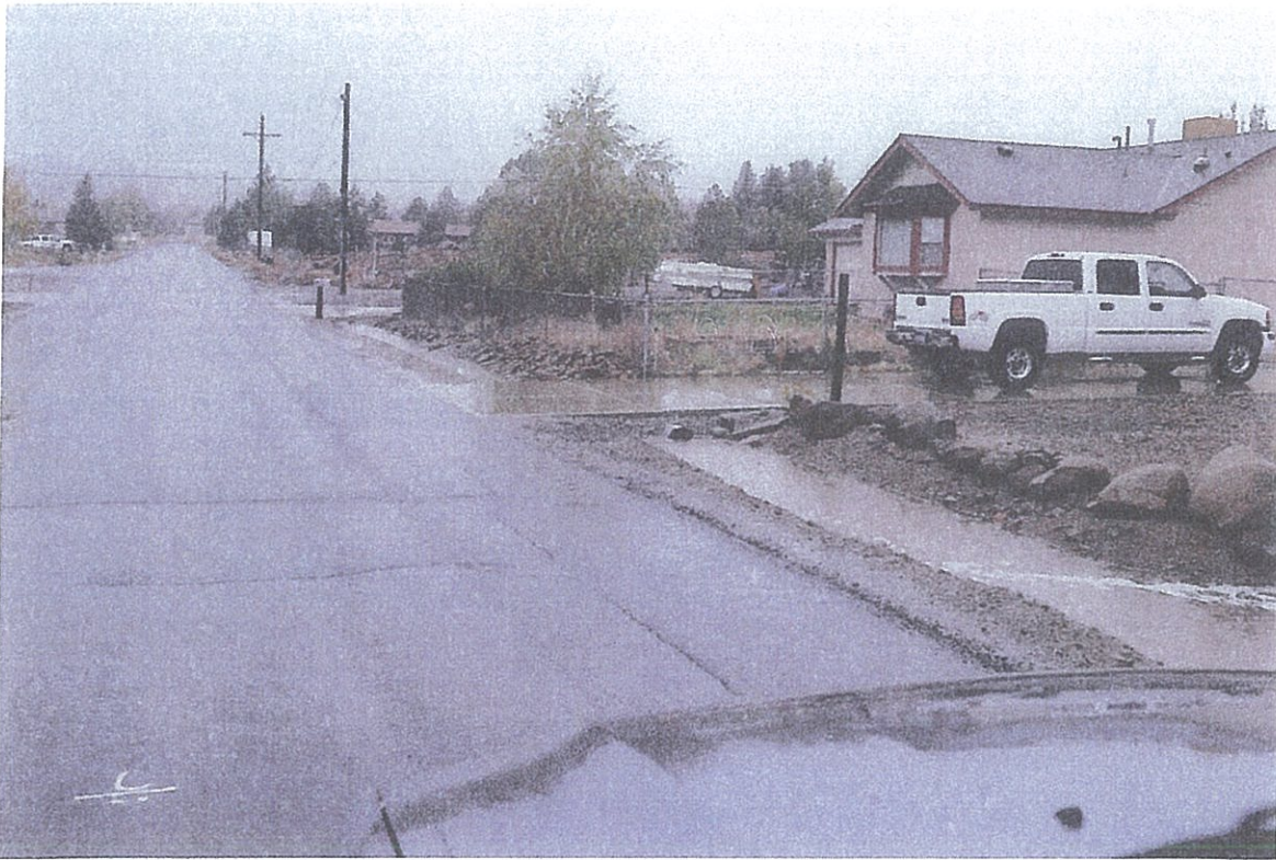
Storm water discharge through a 12" culvert on Shawna Lane. Photograph taken October 16 th 2016 at 2:02 PM.
