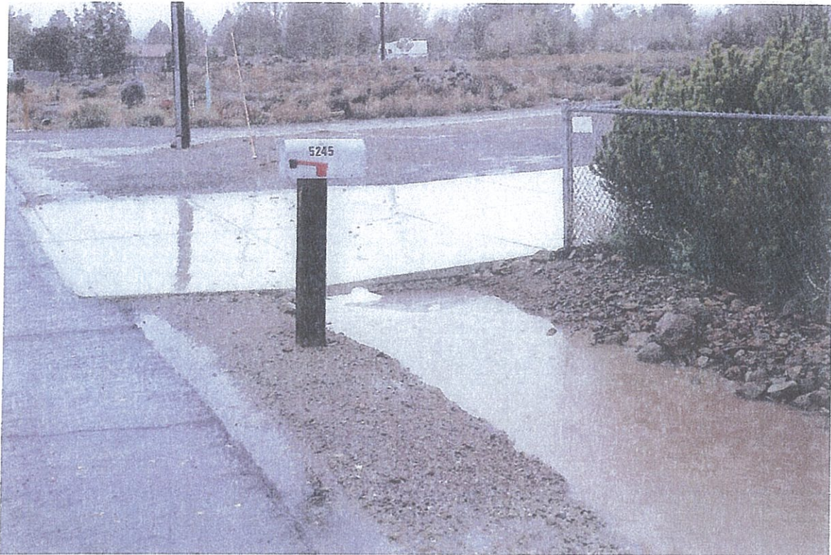
Photograph taken on October 16 th , 2016 at 5:26 PM of 12" culvert on Shawana Lane. Note that discharge is at capacity for this storm water system.
