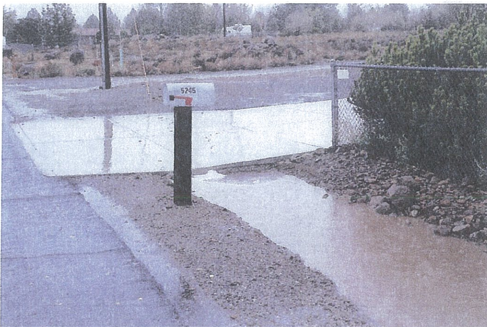
P8. Storm water Flow from the proposed Sierra Village on Shawna Lane. Note that this system is already at capacity. Discharge less than 2 cfs.
