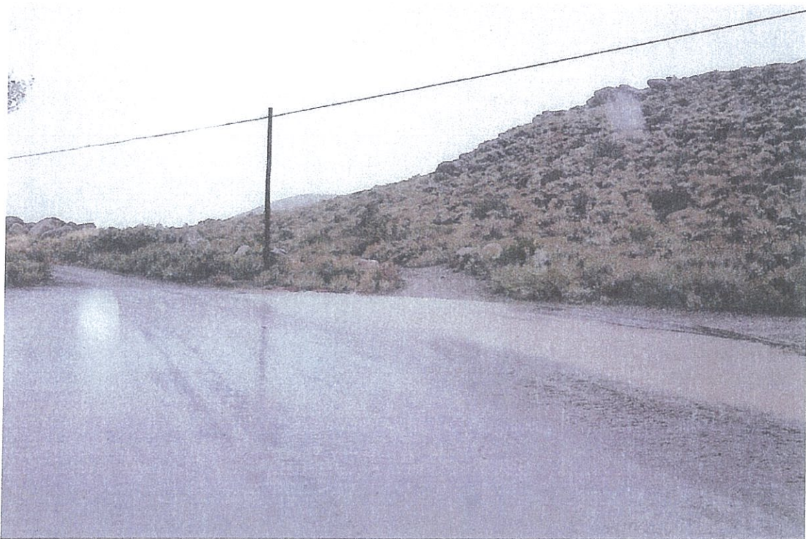
Storm water runoff from area of Sierra Village onto Cedarwood Drive October 16, 2016 2:07 PM.
